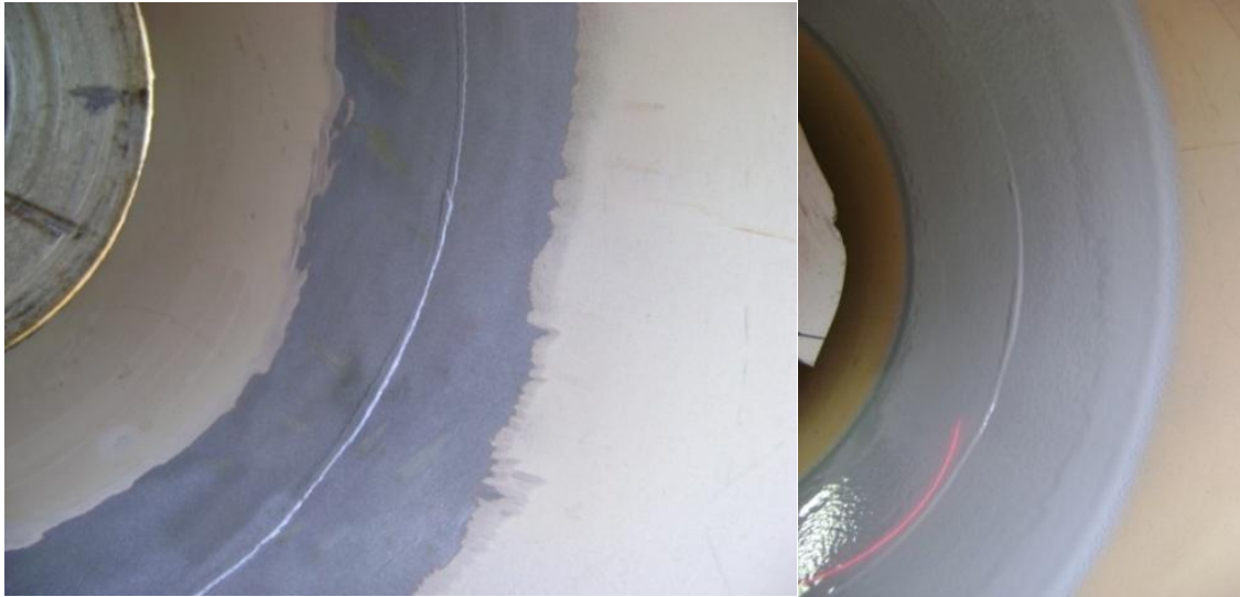
Figure 1. Before and after coating of pipes
