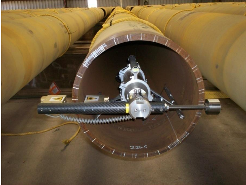
Figure 8. Measurement of 20” pipe ends using the pipe measuring tool
