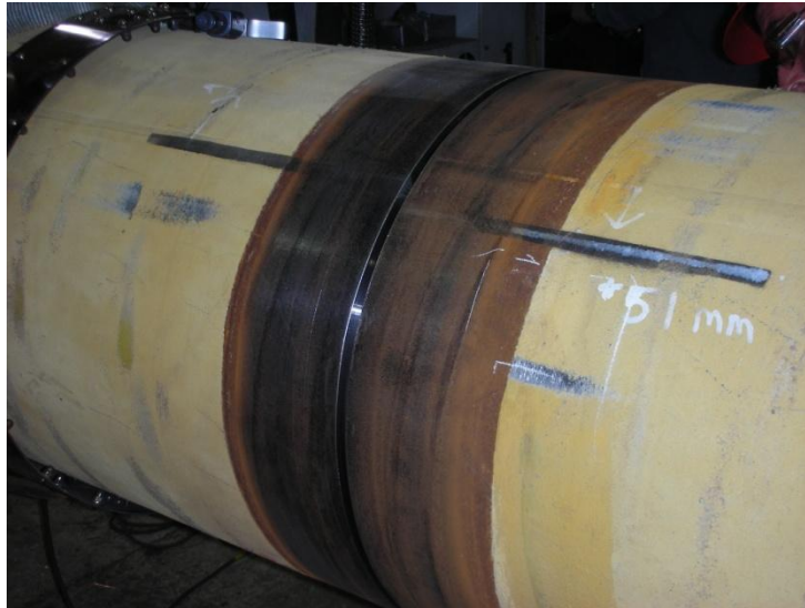
Figure 9. Pipes being rotated into the datum position (both black lines together)
